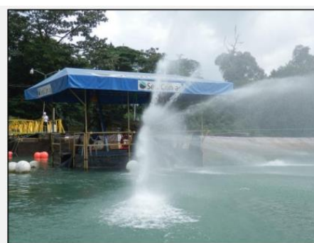
Powerful water jetting disintegrates sediments
